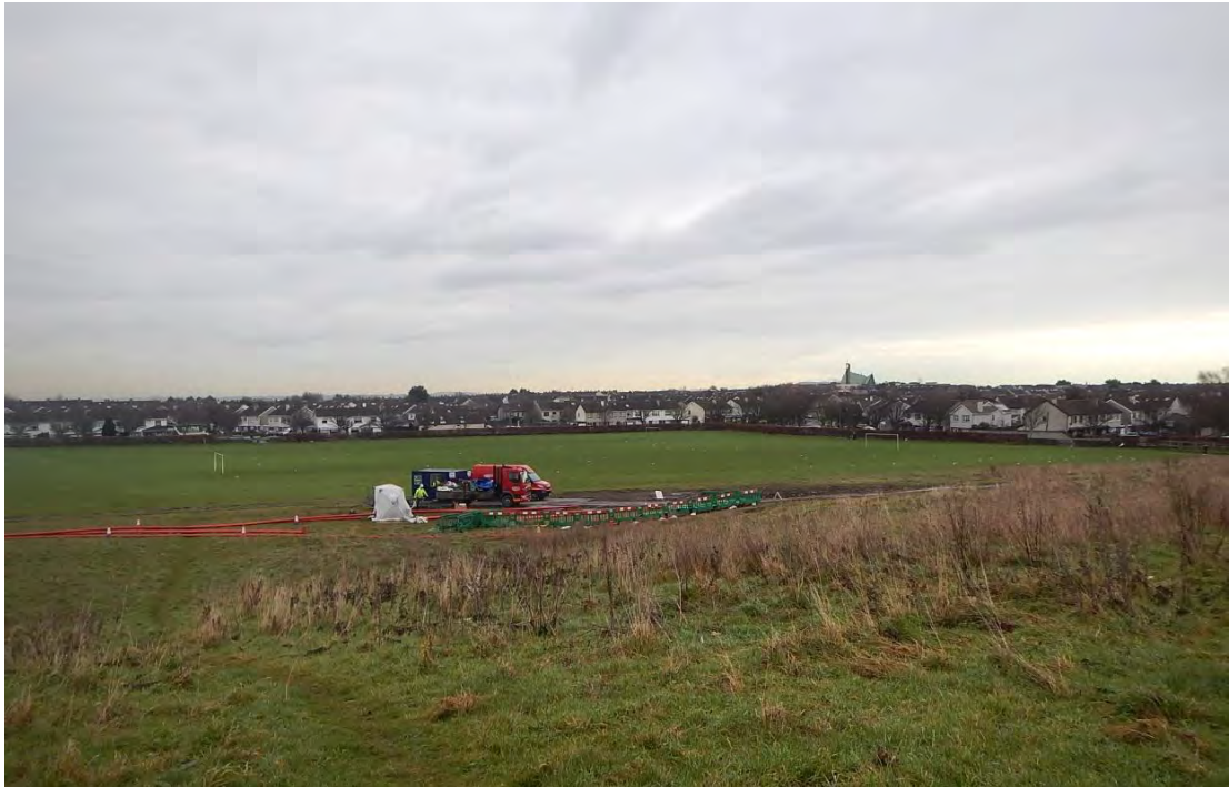
Plate 5. Construction work in a field used historically by brent geese.
