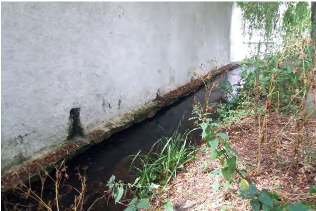
Figure 2. River Poddle at the Poddle Park.
